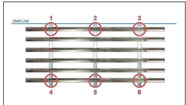
**Step 5:** Fasten remaining horizontal rails.
