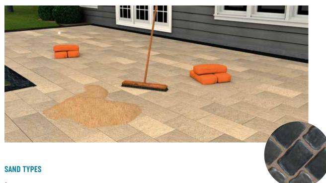
Unilock recommends that you install a jointing sand that conforms to ASTM C936 (semi-coarse sand). Regular sand can be used, but polymeric sand is the most common because it prevents erosion, weed growth and insect infestations. Polymeric sand contains additives that form a binding agent when exposed to water, fusing sand particles together so that pavers are locked in place.
