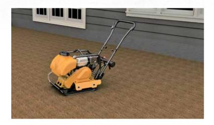
Excavation can loosen the subsoil surface. Before placing any gravel it is recommended that you consolidate the loose surface of the subsoil.
