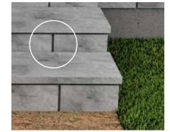
**IMPORTANT:** Sponge off all excess mortar from the surfaces as you go. Wait 2 to 4 hours before adhering the step treads.
