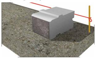
Ensure units are level front to back and left to right. Extra care should be taken at this stage as it is critical for accurate alignment.
