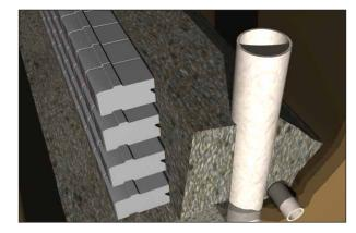
Secure the coping unit and fold filter cloth back over drainage material. Cut filter cloth at centerline of sonotube to allow the sonotube through, ensuring complete coverage of drainage material. Cover sonotubes prior to concrete pour to prevent debris from entering.
