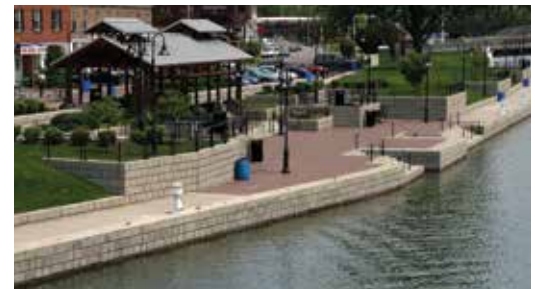
Product: DuraHold2® Project: Erie Canal Location: North Tonawanda, NY Consultant: EDR Consulting
