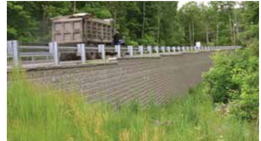
Product: Pisa2/Concord Wall™ Project: Roadway Retaining Wall Location: Uxbridge, Massachusetts Consultant: Risi Stone Systems
