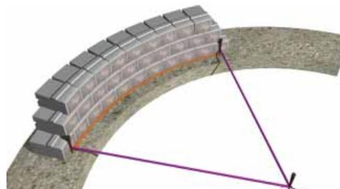
Geogrid layers should be placed within 25mm (1 in) of the front face of the block. It will be necessary to have gaps between adjacent sections of geogrid. At alternating geogrid elevations the geogrid sections should be positioned so they overlap the gaps in the geogrid on the layers below.
