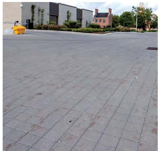
Rust marks on pavers from metal blade plow
