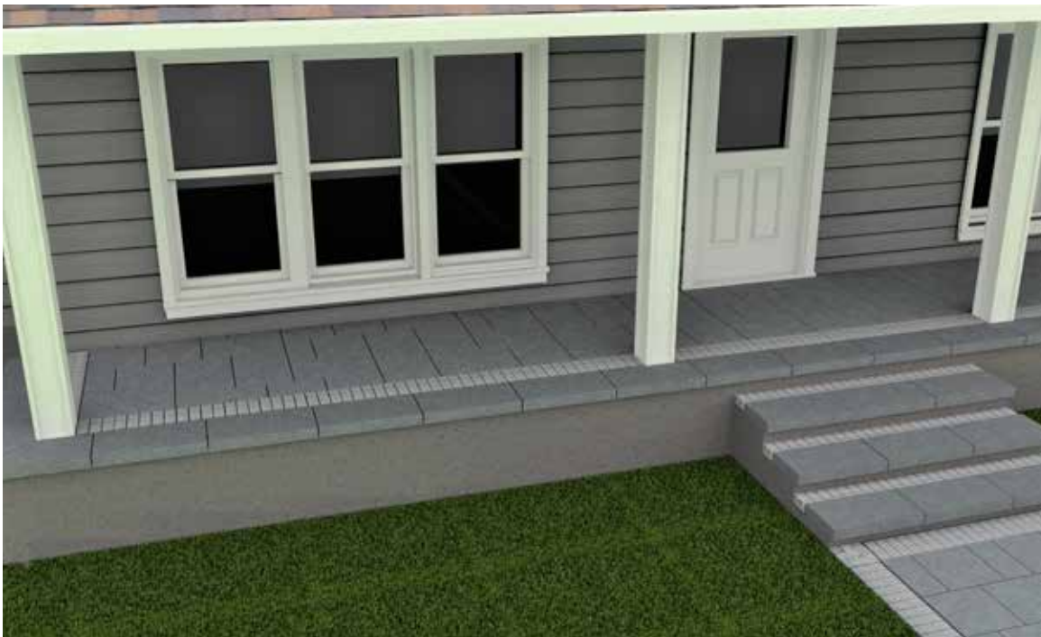
Completed Porch Overlay with Paver
