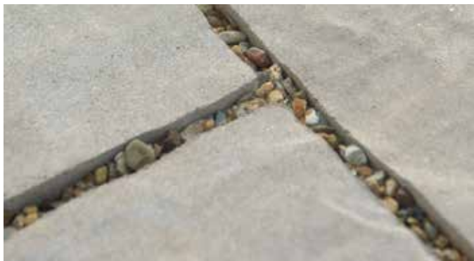
Special materials are used in the joints and in the permeable base below, to encourage water to flow through.
